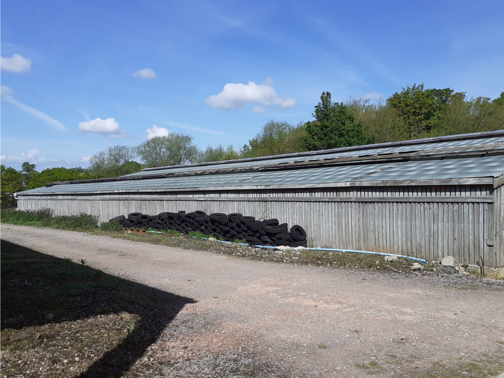
South (front) elevation of Building C
