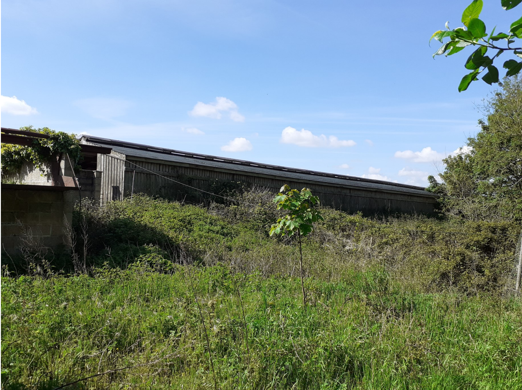
North (rear) elevation of Building C
