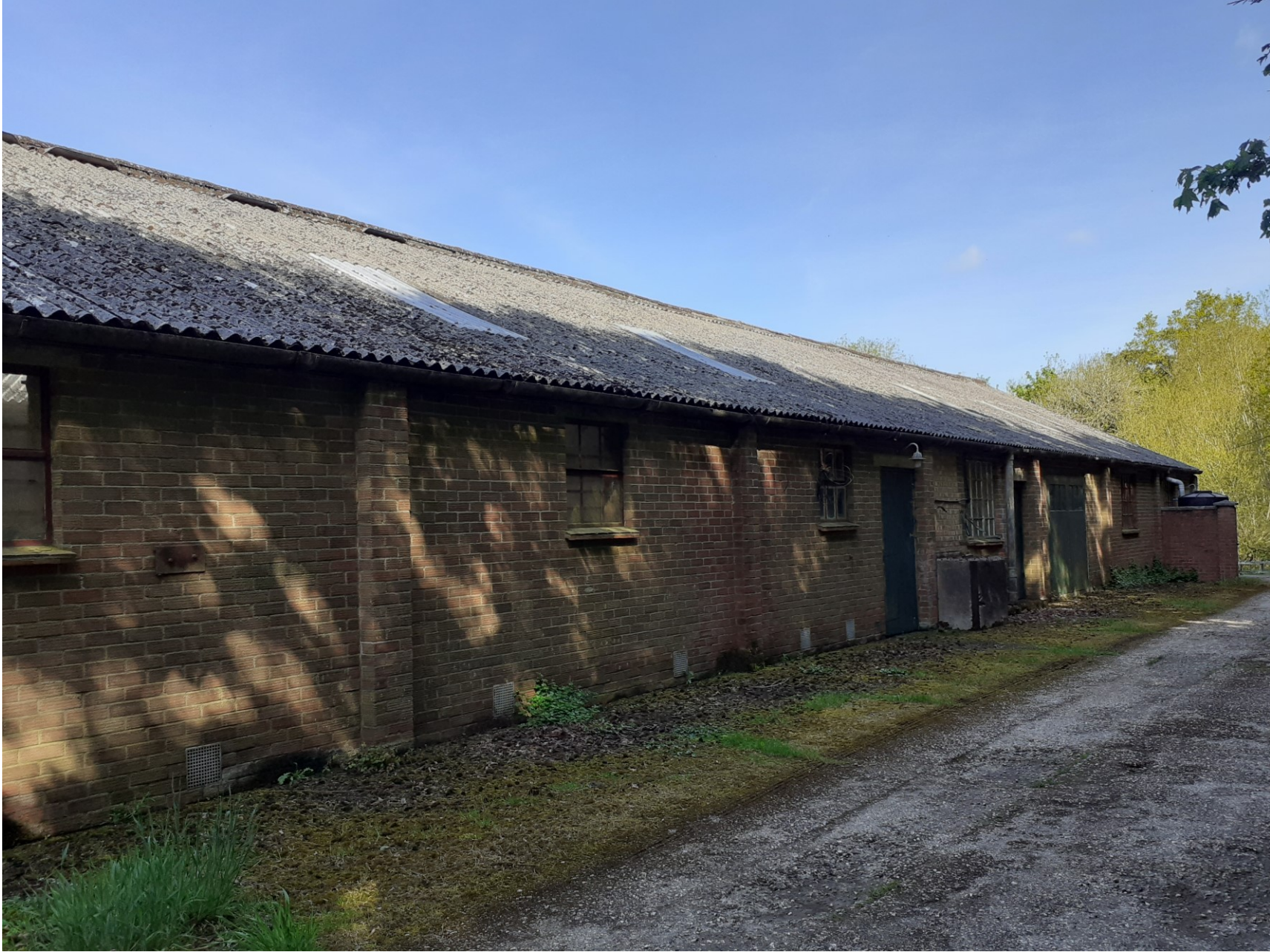
Rear (east) elevation of Building A
