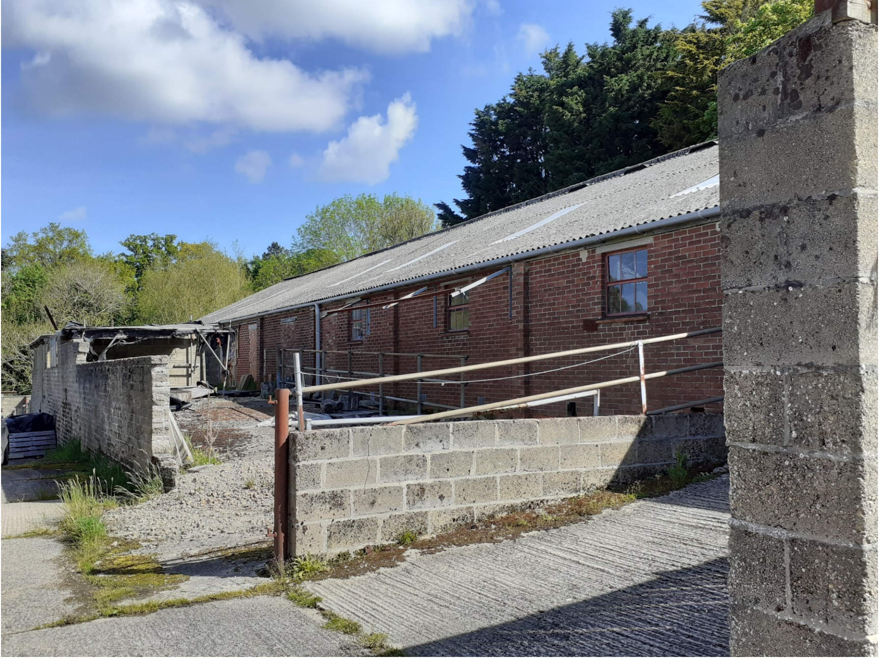
West (front) Elevation of Building A
