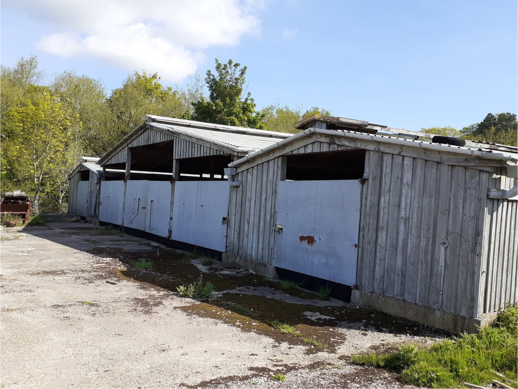
Side (west) elevation Building C
