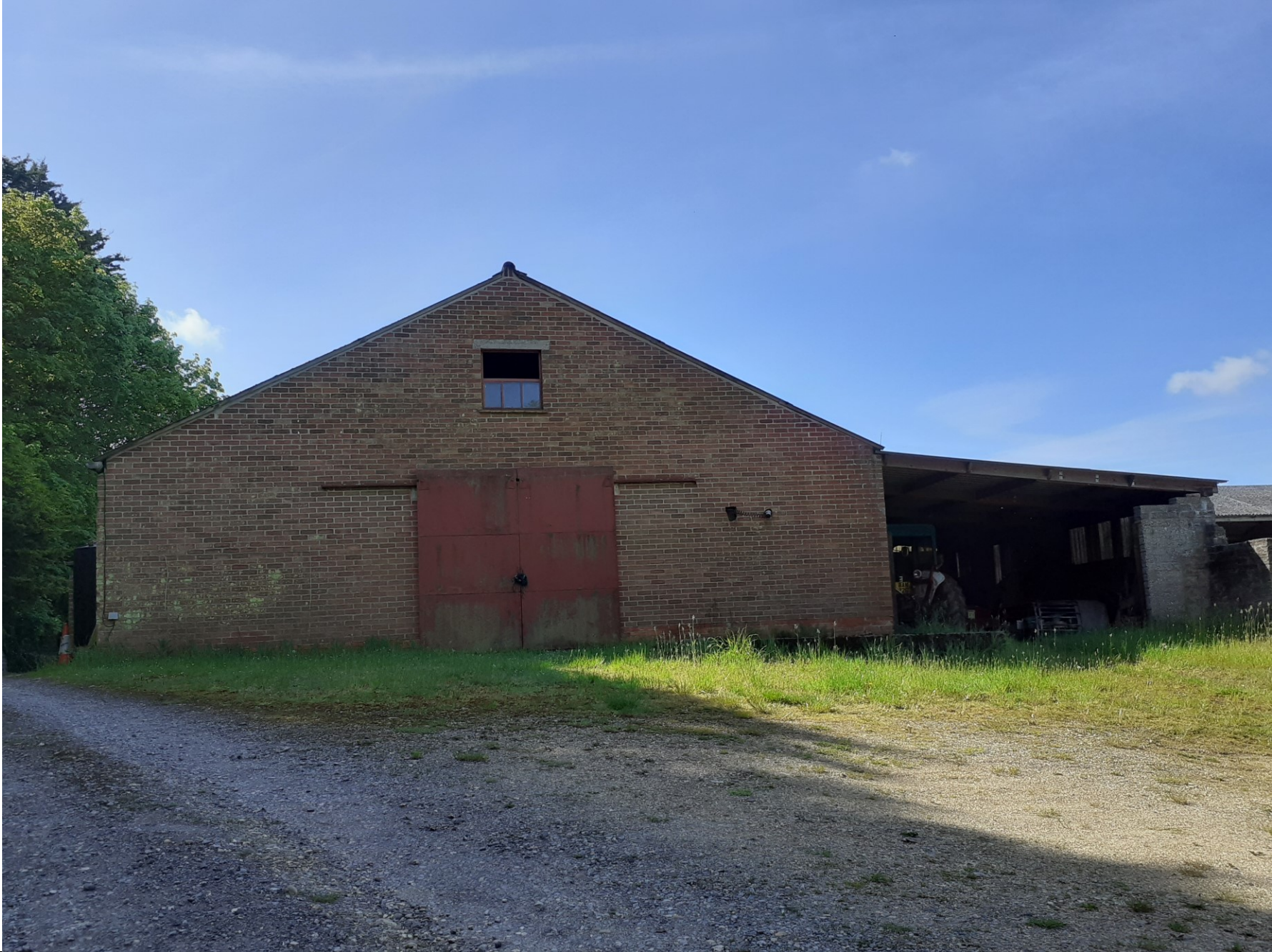
Northern elevation of Building A
