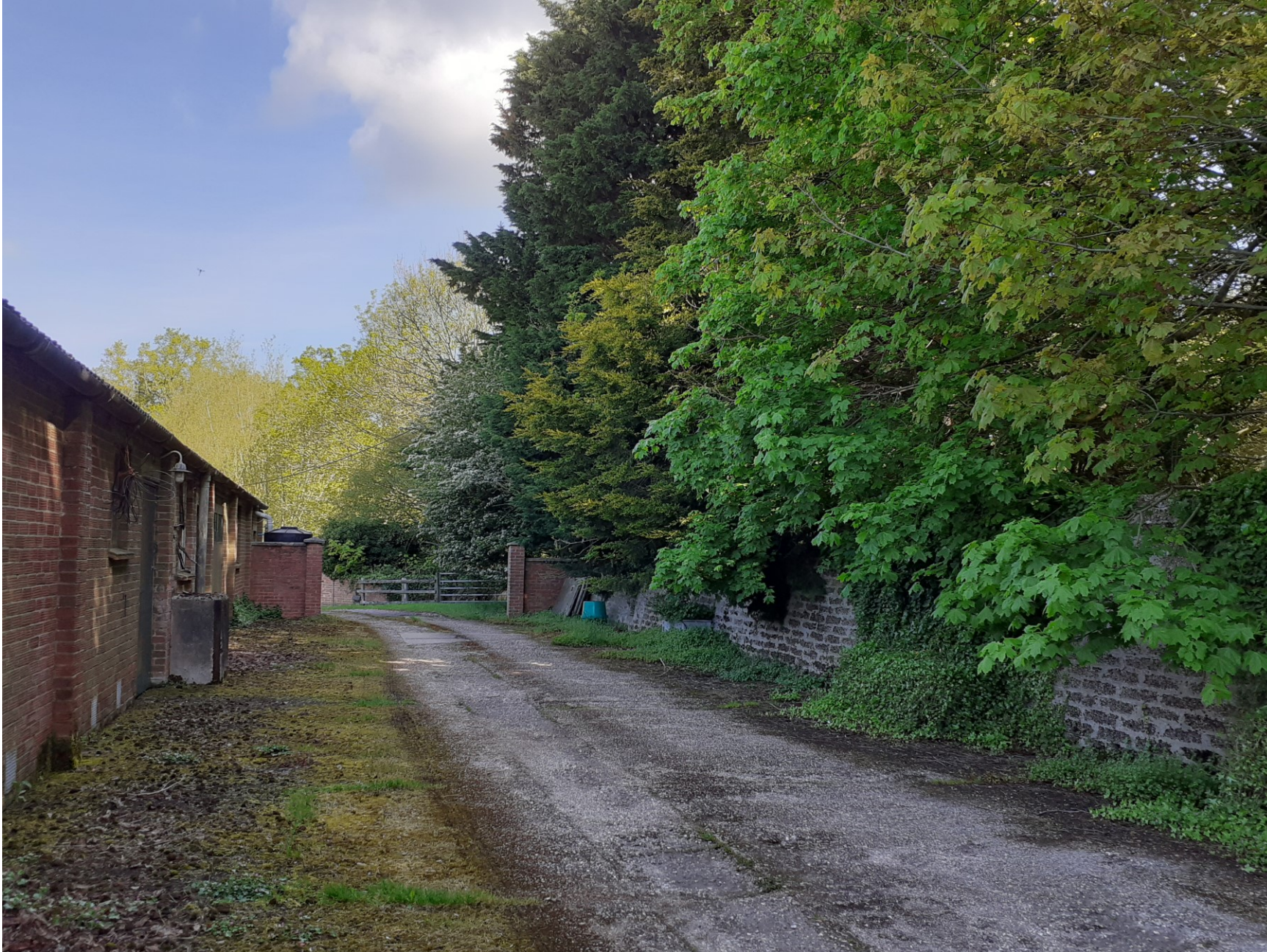
Rear (east) elevation of Building A and eastern site boundary
