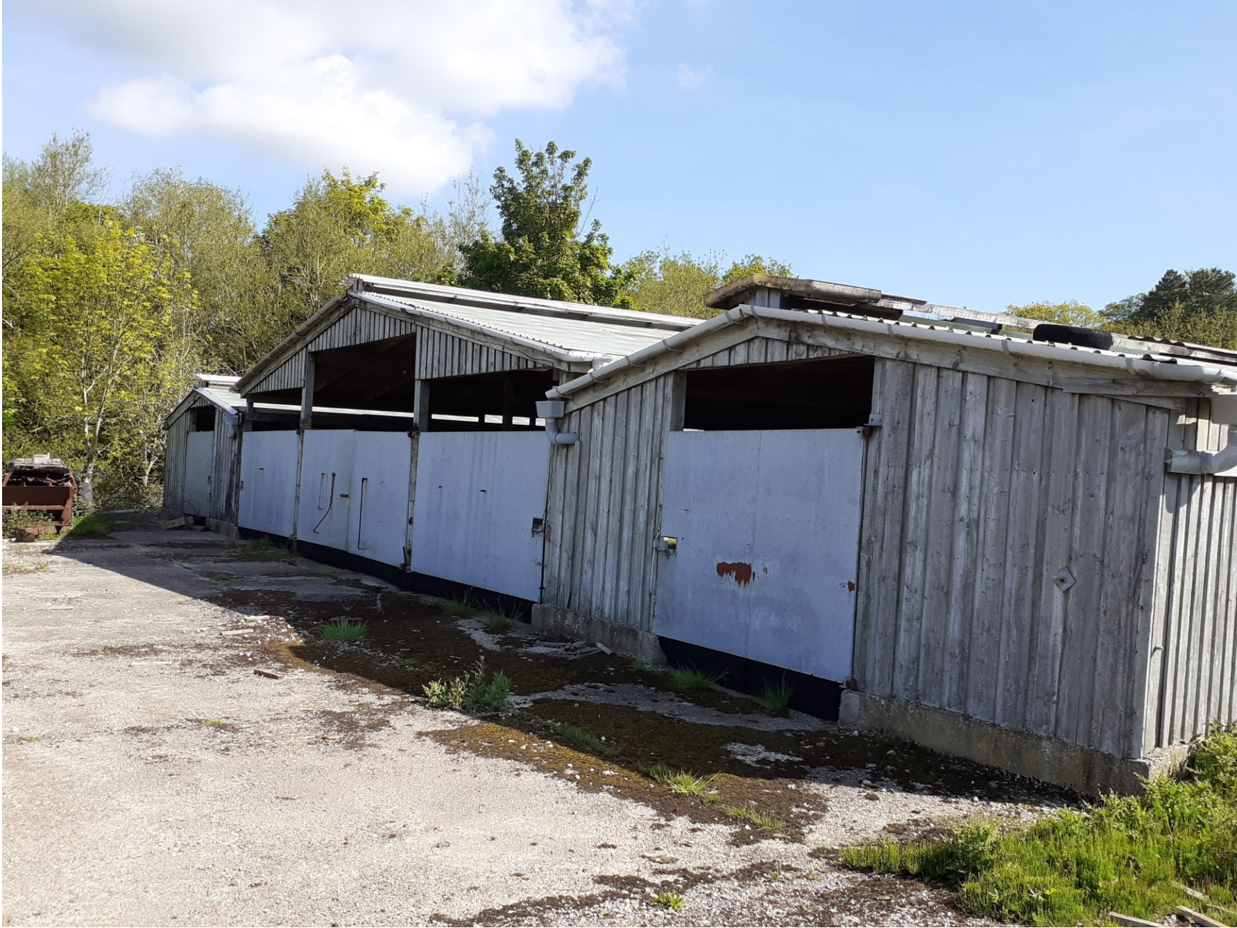
Side (west) elevation Building C
