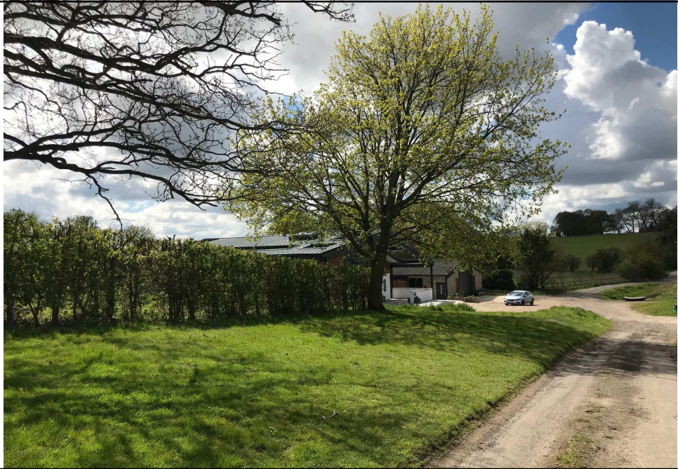
View of site from byway to the north
