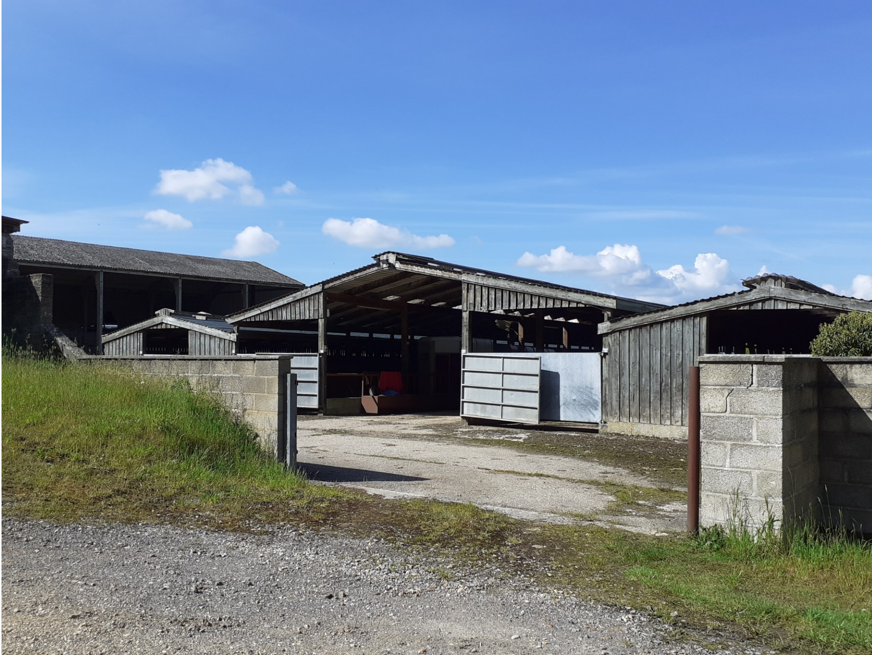
Side (east) elevation of Building C
