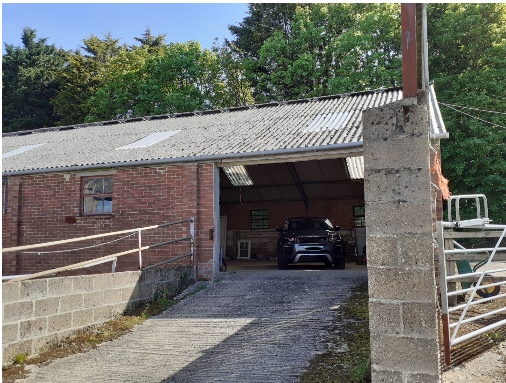
West (front) elevation of Building A
