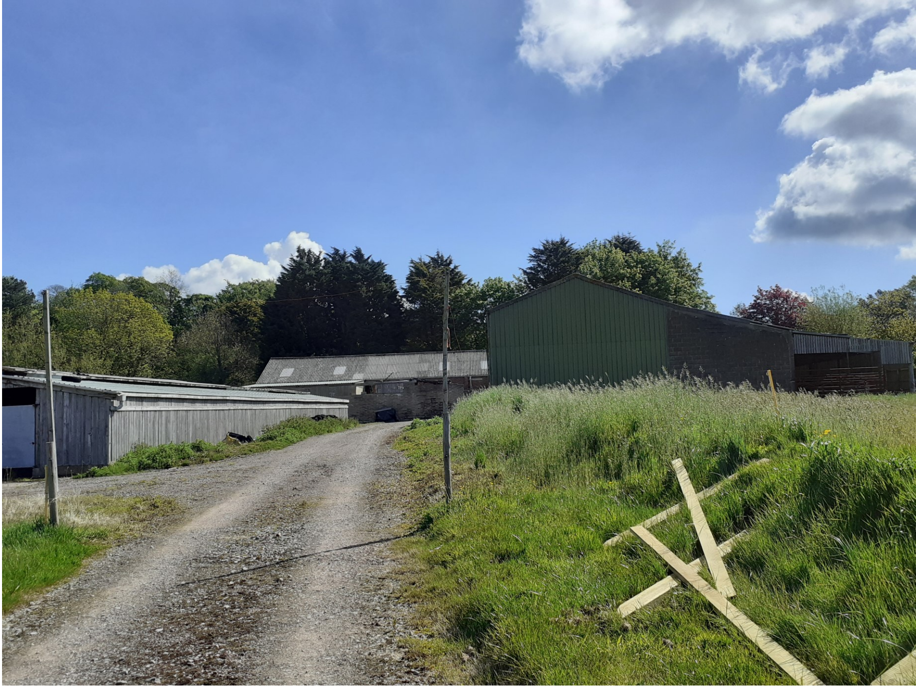
Building C south elevation, Building A west elevation and Building B (to be demolished)
