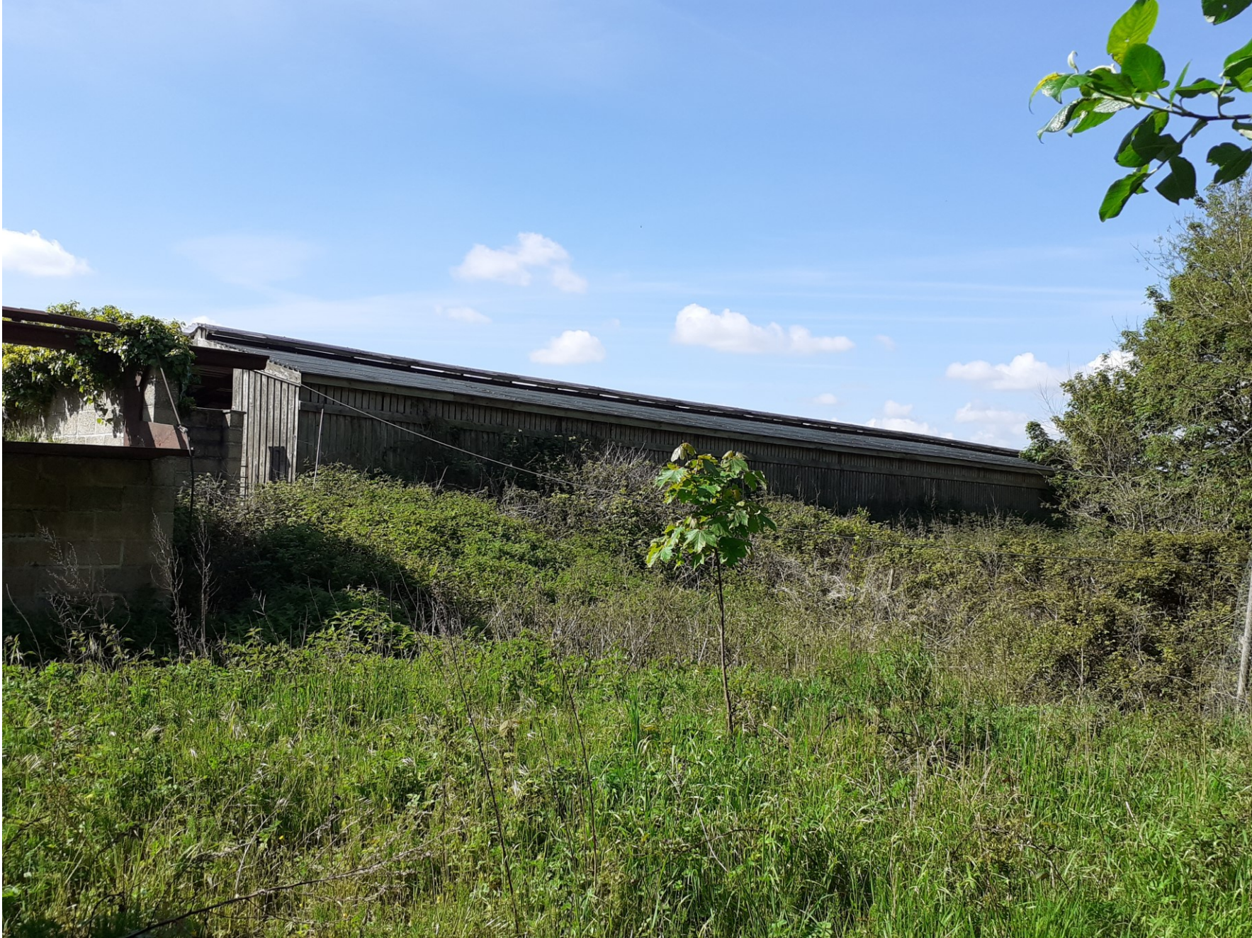
North (rear) elevation of Building C
